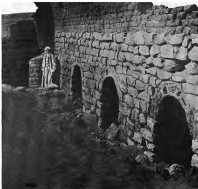
(a) Interior looking west, before excavation.
